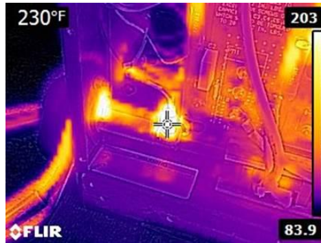
Demonstrates excessive heat at a loose connection on a welder repair.
